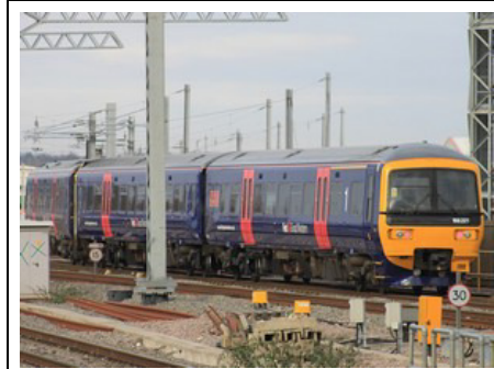
RIGHT BEHIND CARDIFF ROAD: a train at the new depot (Photo: Geof Sheppard)
